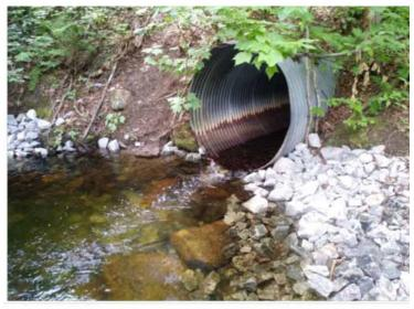
Figure 3: Upgrading of a pipe downstream of a culvert on the Éternité River allowing access to the American eel. Photo: Akian Gros-Louis Picard
